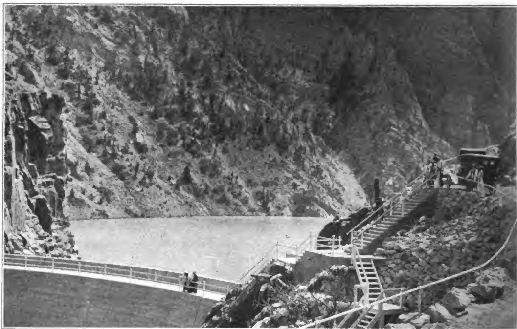
THE SHOSHONE DAM, CODY, WYOMING—ONE OF THE FACTORS WHICH IS RAPIDLY CHANGING THE OLD COW-COUNTRY INTO AGRICULTURAL AREAS. THIS DAM IS 329 FEET HIGH AND FORMS A LAKE 18 MILES LONG AND SEVERAL MILES WIDE.
